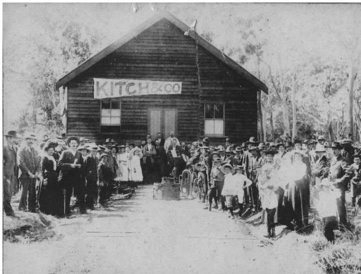
Opening of the School of Arts, 16 August 1904, Picture Coffs Harbour Museum 07-1430
